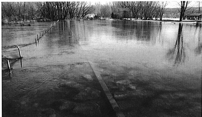
Figure 6-2 Stone Weir just after construction – 1999
