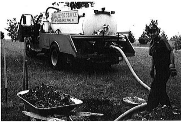
Pumping your septic system every 3-5 years increases the life-span of the system.
