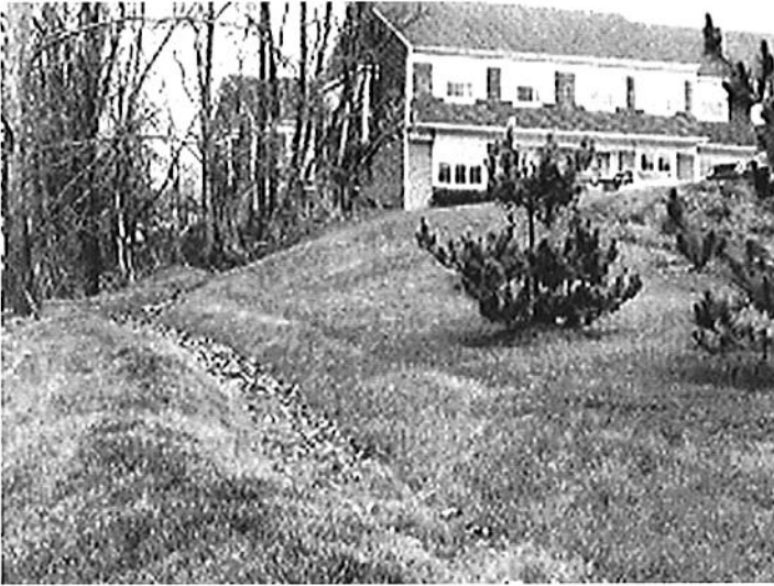
An example of a swale—intercepts runoff and controls erosion across a steep slope.
