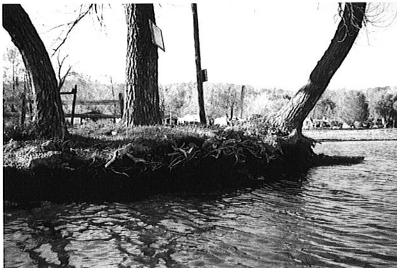
Shoreline Erosion along west side of lake
