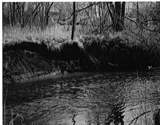
Stream banks are eroding due to flows and lack of vegetation.
