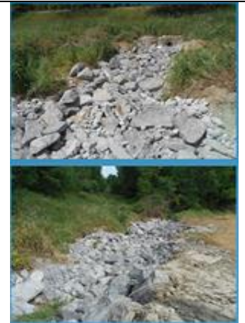
Right: Rock armoring of erosion prone streambank at Muller Field Station
