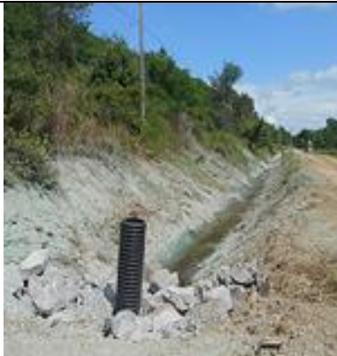
Left: Water Control Structure at Muller Field Station: Improved drainage swale & standpipe control completed
