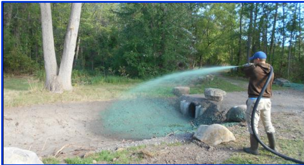
Photograph: Megan Webster: Tucker Kautz hydroseeding at Sandy Bottom Park drainage project.
