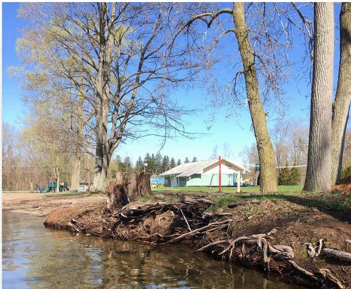
Coir wrapped soil lifts that incorporate native plant materials were utilized to reconstruct the eroded bank. Existing tree and shrubs were
